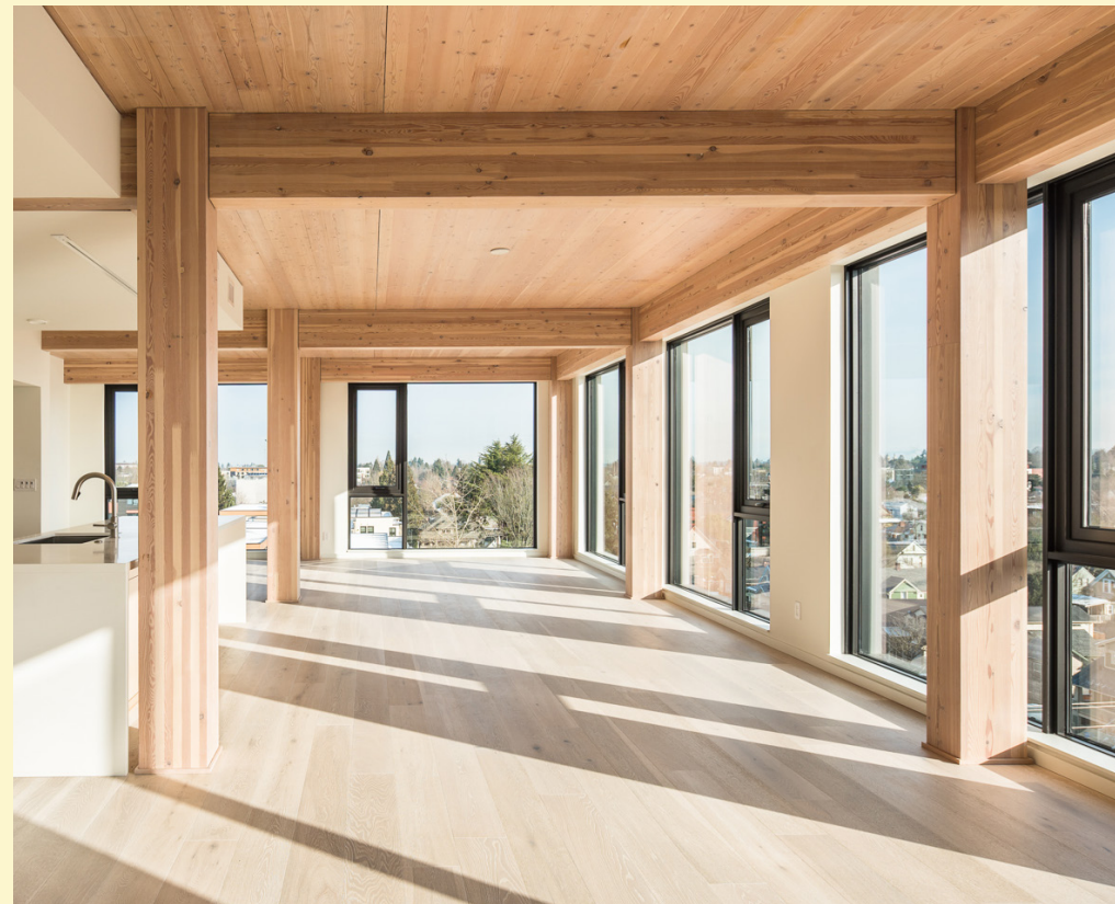
← Carbon 12, Portland, Oregon by Kaiser + Path This 85-foot-high mass timber condo provides residents with modern luxury, sustainable design and state-of-the-art technology. Constructed with sustainably harvested and certified CLT, when it was completed in 2018 it was one of the tallest buildings of its kind in North America, and the project is opening the doors to taller wood buildings throughout the state. (c) Andrew Pogue
